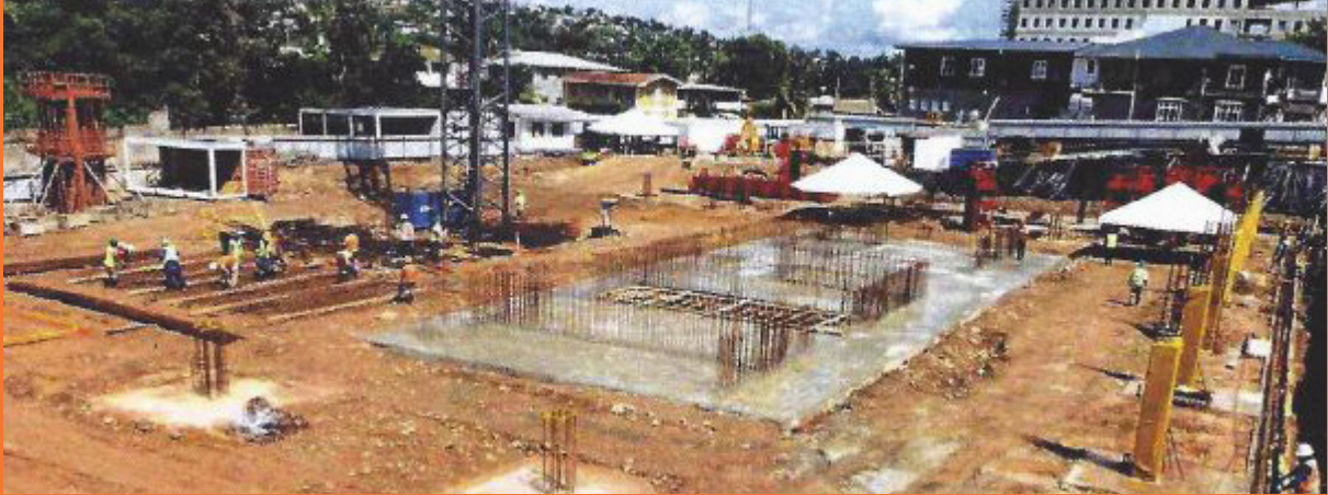
Concrete Raft Foundation July 2015.
